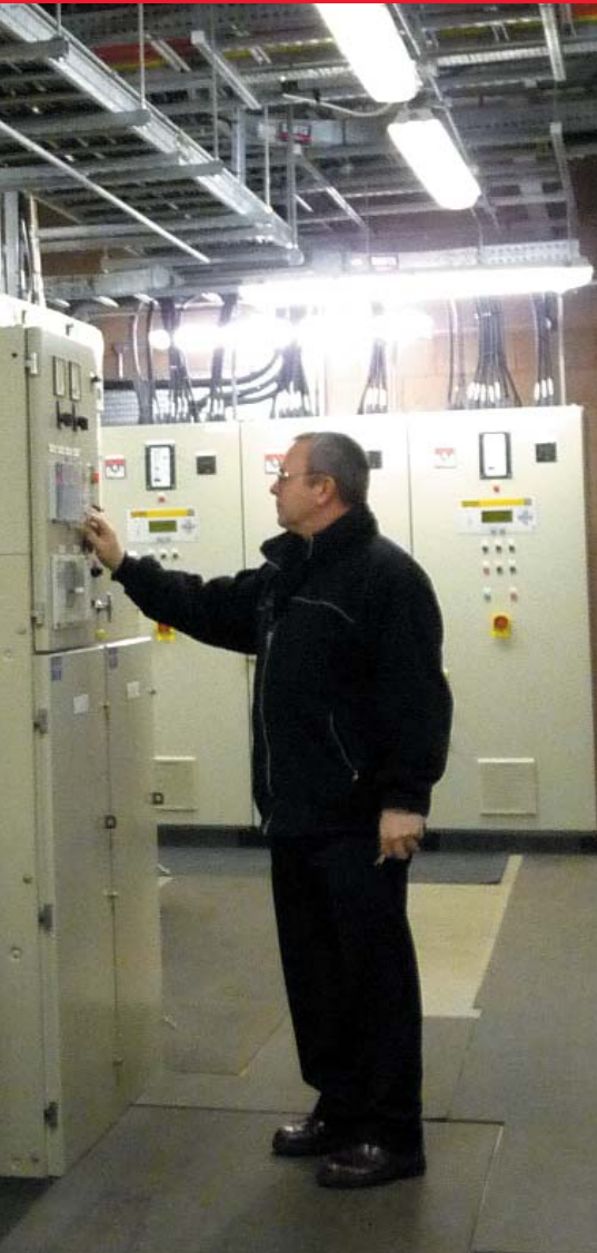
The four NNUH generators are controlled through a series of complex circuit boards (far left), while the generator engines (left) are housed in separate metal containers in the hospital grounds
