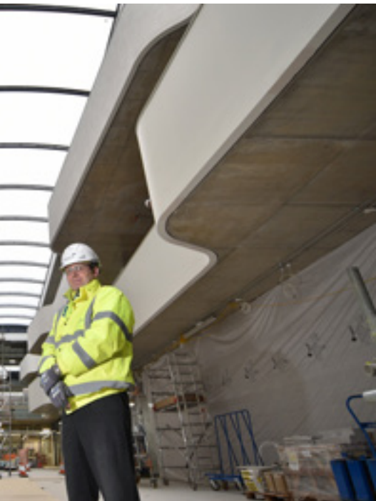
Simon Rushbrook and Waites Project Director, the new Quadram Insitute Building CREDIT: EDP/ANTONY KELLY
