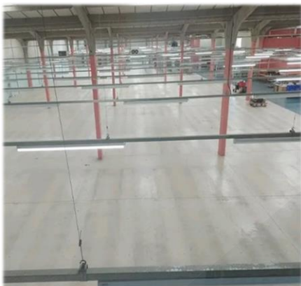
The former HRL at Francis Way being cleared for the move
